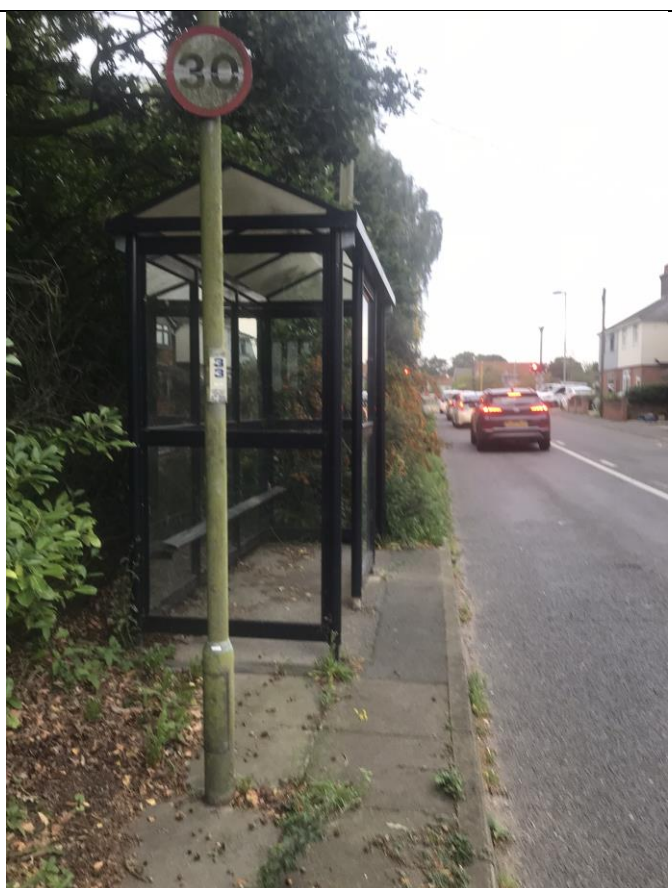
Lack of pavement from Bus Stop to Station
