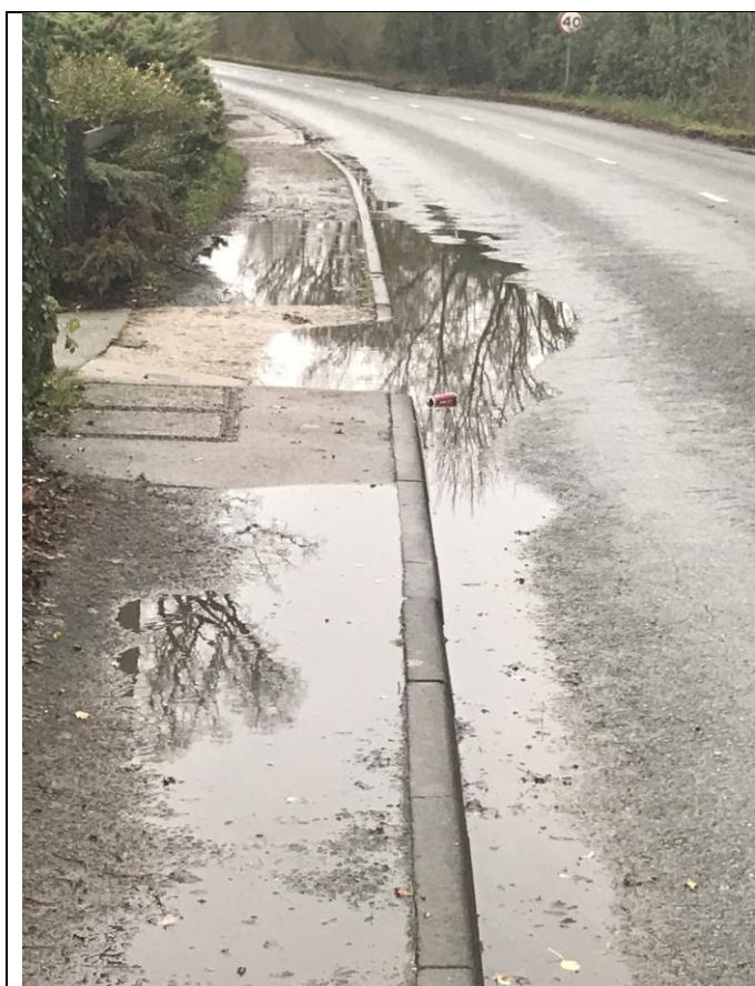
Pavement to south of Westerfield Station
